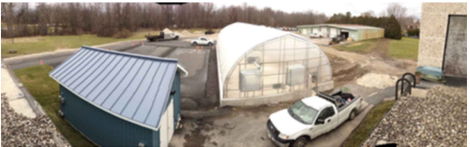
Completed Perth Residuals Treatment Facility
